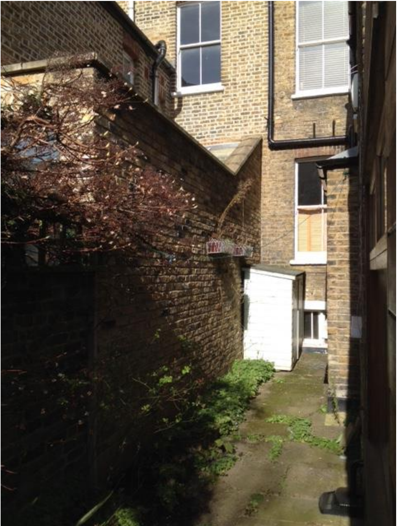
Image 4 – View of existing extension on neighbouring property
