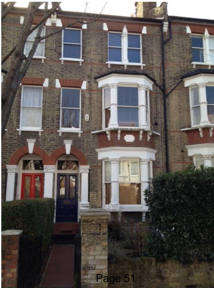
Image 2 - View of front elevation
