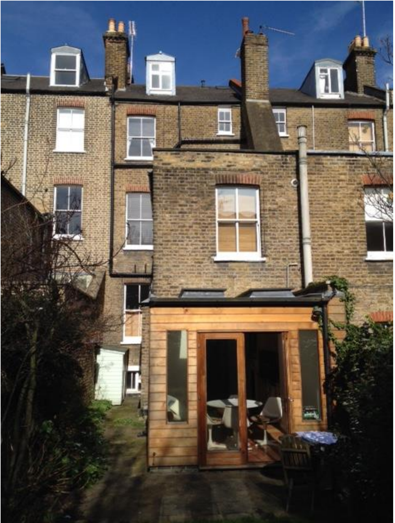
Image 3 – View of Rear Elevation
